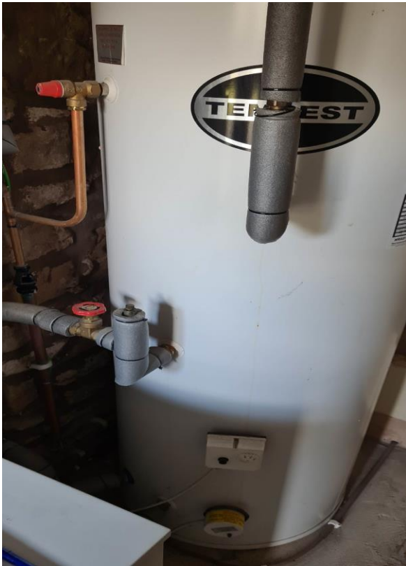
Old Walls Calorifier
